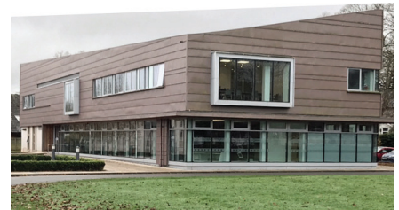
Current Canterbury Building, courtesy of Esther Weller, November 2021
