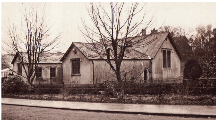
From a postcard (courtesy of Richard Morton) which probably dates from before World War I. An unprepossessing winter view of the College School looking from an unmade Station Terrace. In the background above the school is Springfield (after Wycliffe College's Springfield House), which took over what had been Professor Hugh Walker's old home in WW II – he had died in June, 1939. Springfield was demolished in 1967 to make way for Lloyd Thomas Hall.
